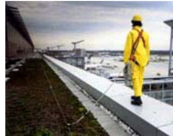
This worker is protected by a properly constructed fall arrest system.
