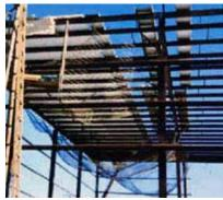
A safety net is being used under the roof of this building as an acceptable fall protection system.
