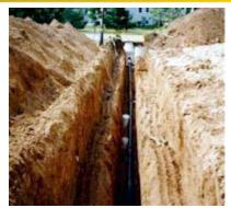
The spoil pile is required to be at least 2 feet from the edge of the trench and/or retained to prevent it from falling into the trench.
